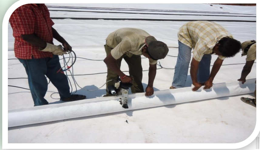
LATERAL PIPE LINE RAPING WORK
