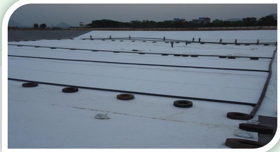
HDPE LEACHATE PIPE LINE NETWORK
