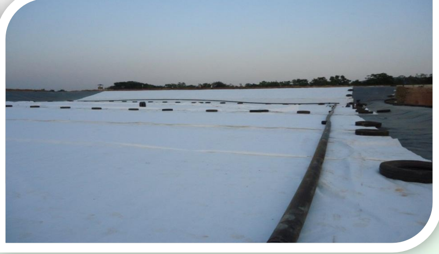
400 GSM GEO TEXTILE LAYING
